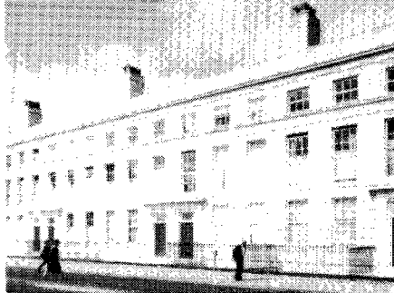
Constructed 36 flats for the Young Persons Housing Association
