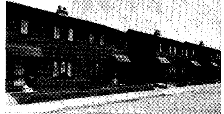
Designed and built 29 Homes for Liverpool City Council
