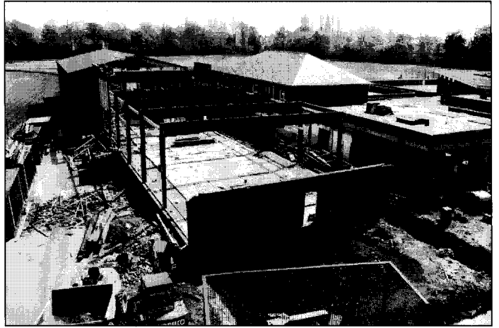
The new dining room taking shape as work gets underway
